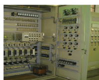
PLC制御盤 PLC Control Board
