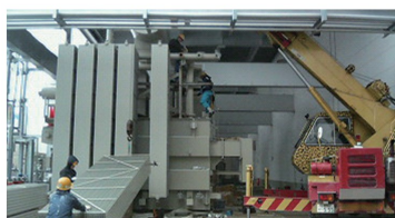
■変圧器(乾式／油入)の組立・保守 Assembly and Maintenance of (Dry / Oil-Filled) Transformers
